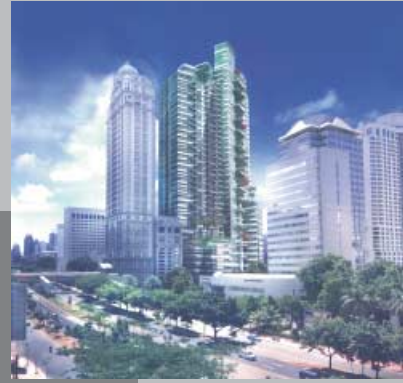
■ Sahid Sudirman Residence, Jakarta Sahid Sudirman Residence, Jakarta
