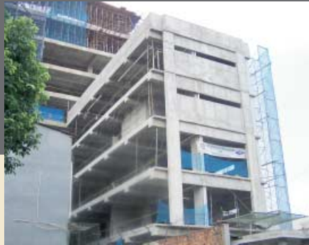
■ Konstruksi Bangunan Prodia Tower, Jakarta Prodia Tower Building Construction, Jakarta
