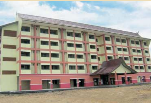
Rusunawa, Banjarmasin Precast Building Element and Precast Contractor by PT Pacific Prestress Indonesia
