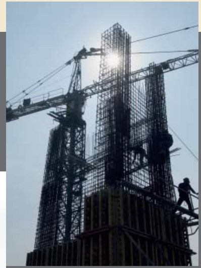
■ Konstruksi Bangunan Thamrin Nine, Jakarta Thamrin Nine Building Construction, Jakarta
