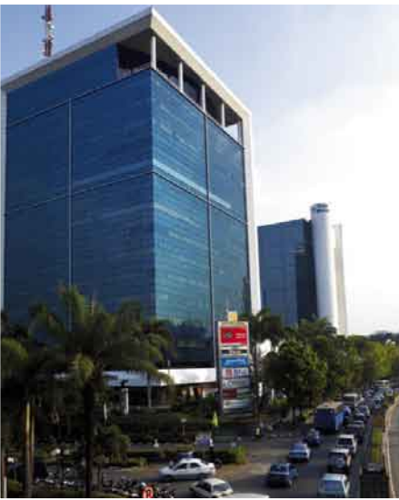
Graha Surya Internusa Office Building
