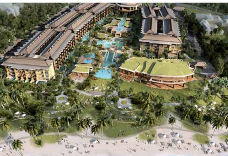
NRCA Project - Sofitel Luxury, Bali
