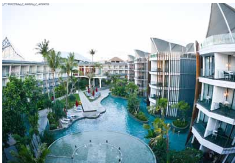
NRCA Project - Le Meridian Jimbaran Bali
