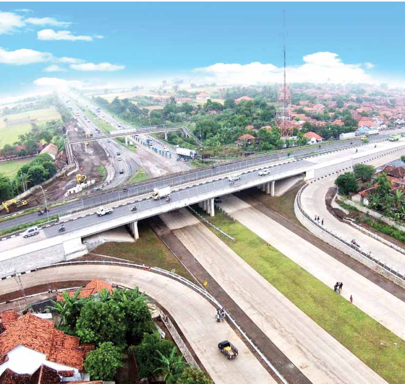
NRCA's Project: Proyek Jalan Tol Cikampek-Palimanan 116 Km
