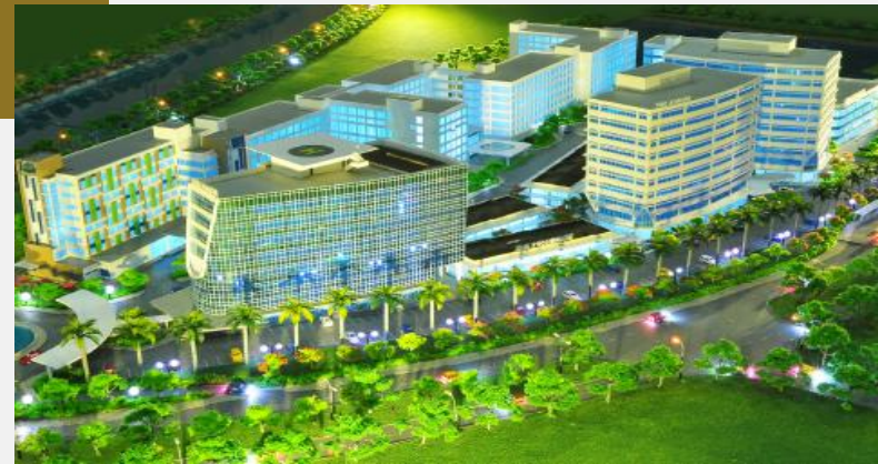
Commercial Area Development
