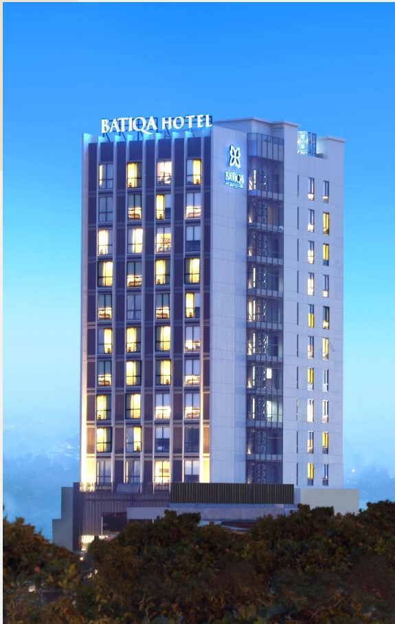
Exterior view of BATIQA Hotel Lampung
