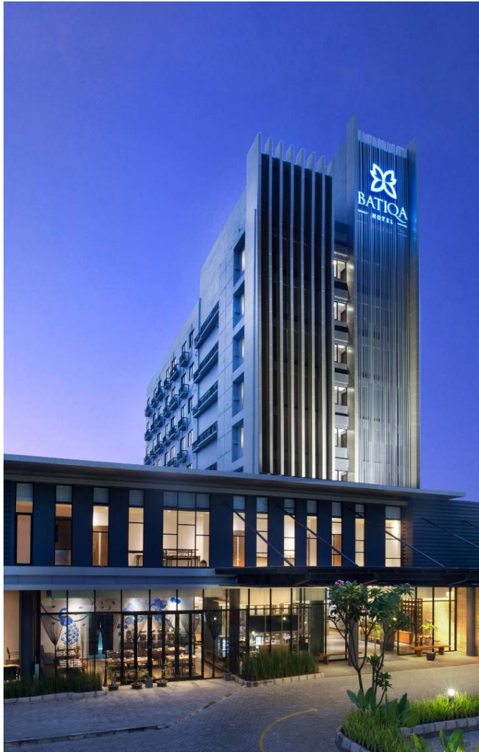
Exterior view of BATIQA Hotel Cirebon
