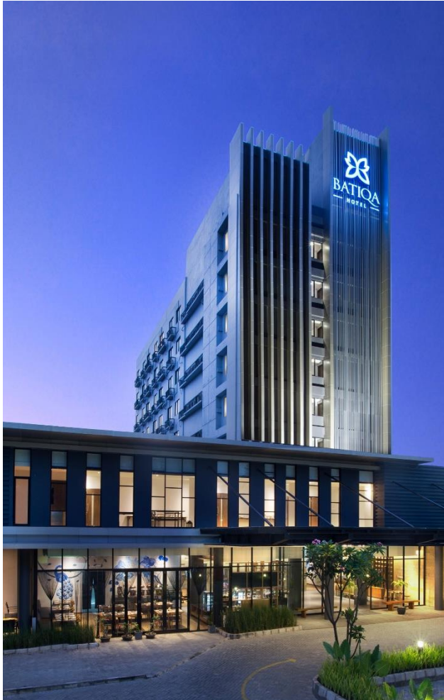
Exterior view of BATIQA Hotel Cirebon
