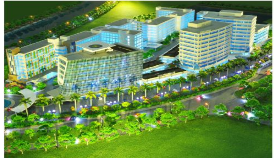
Commercial Area Development
