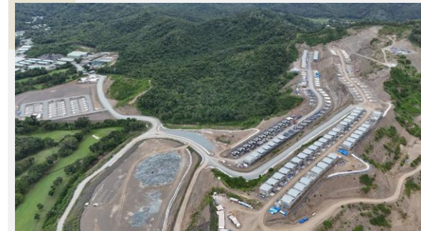
New Townsite Amman Mineral – West Nusa Tenggara
