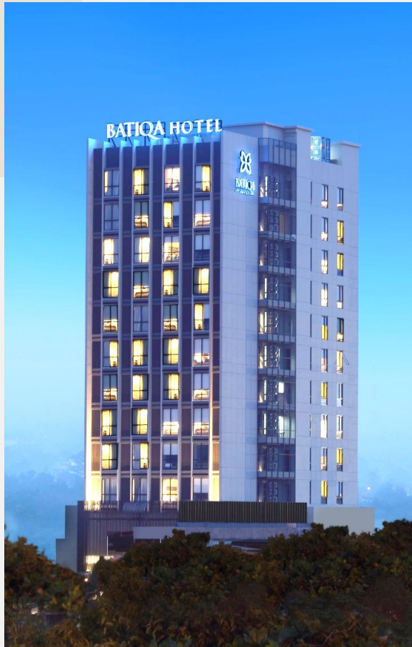
Exterior view of BATIQA Hotel Lampung
