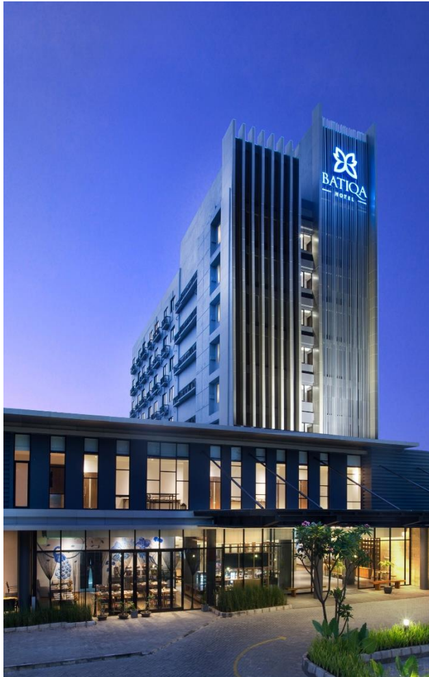
Exterior view of BATIQA Hotel Cirebon
